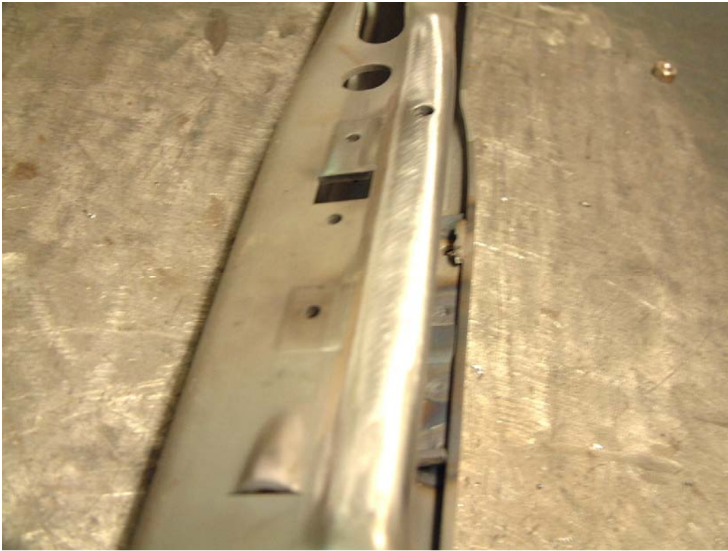
19- Grind welds flush and smooth.
